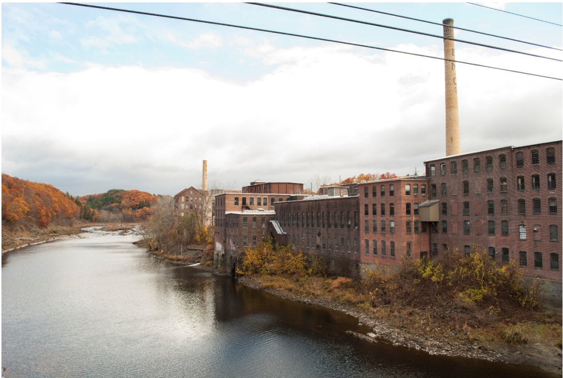
Figure 18: View of the west side of the Power Island Mill
