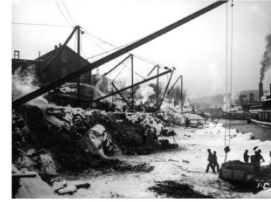
Winding of the Power Canal Source: The Planning and Development of Forest Hills, Massachusetts
