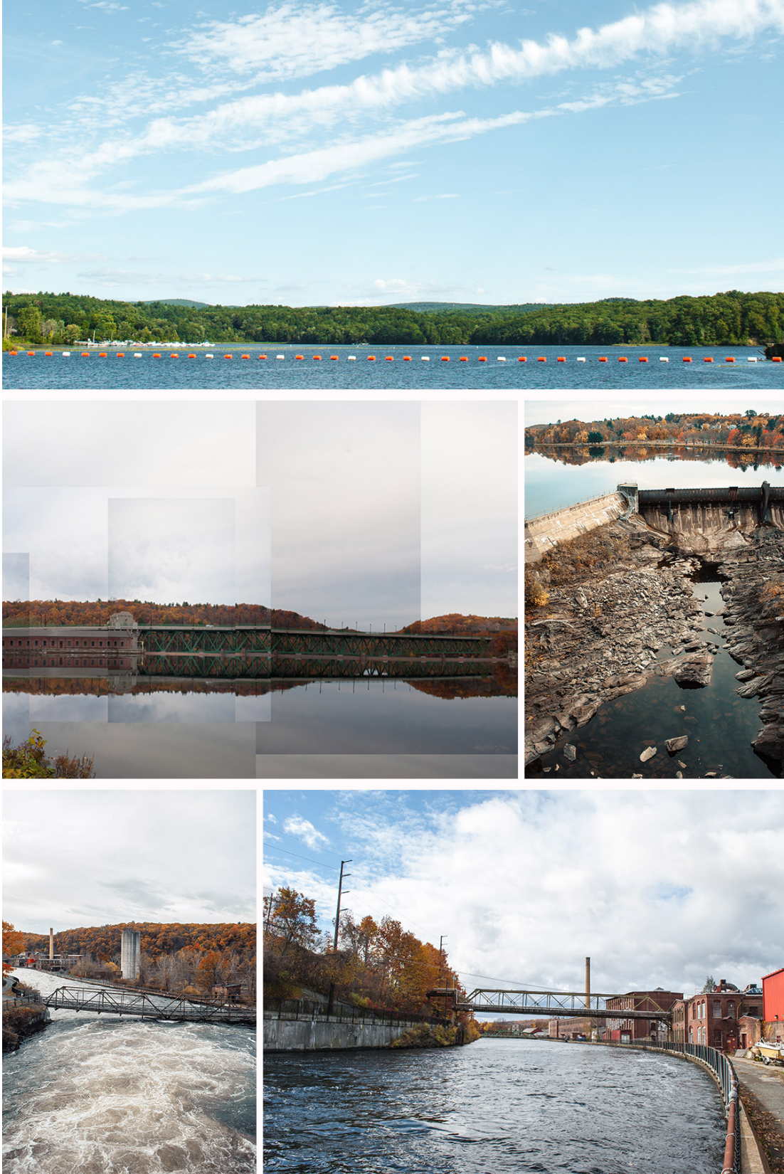
Figure 17: A visible dichotomy of experience and spatial quality above and below the Turners Falls Dam
